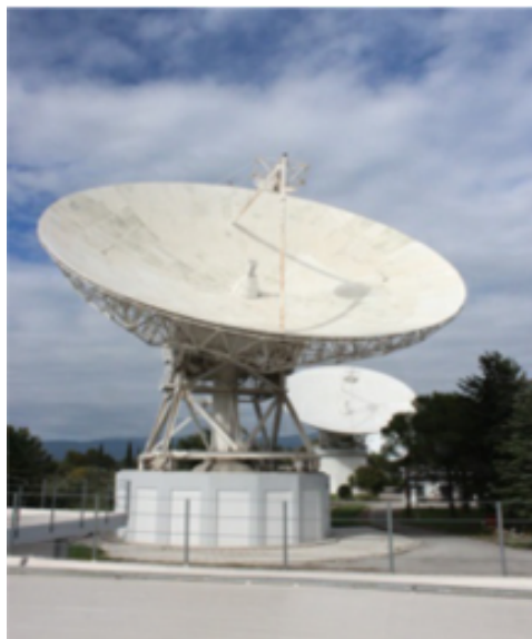
Figure 9. Photo of the C-band Satellite Telecommunications Antenna (photo credit K. Papathanasopoulos)
