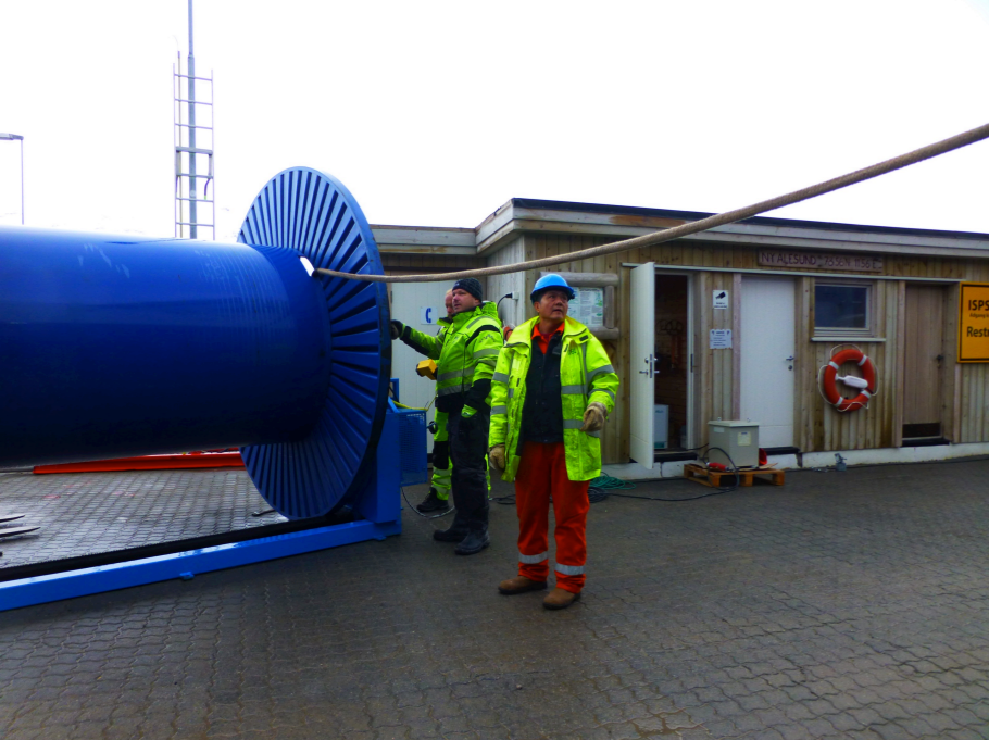
offloading spare cables (2x 5km over to drums)
