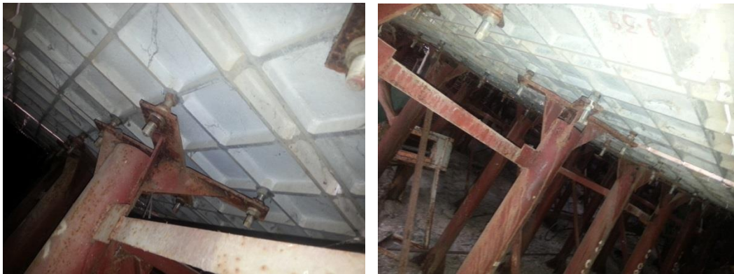
Fig.3 Panel mounting, Average gap width between panels indicated as 2 mm.
