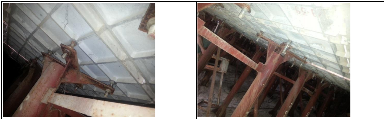
Fig. 3 - Panel mounting, Average gap width between panels indicated as 2 mm
