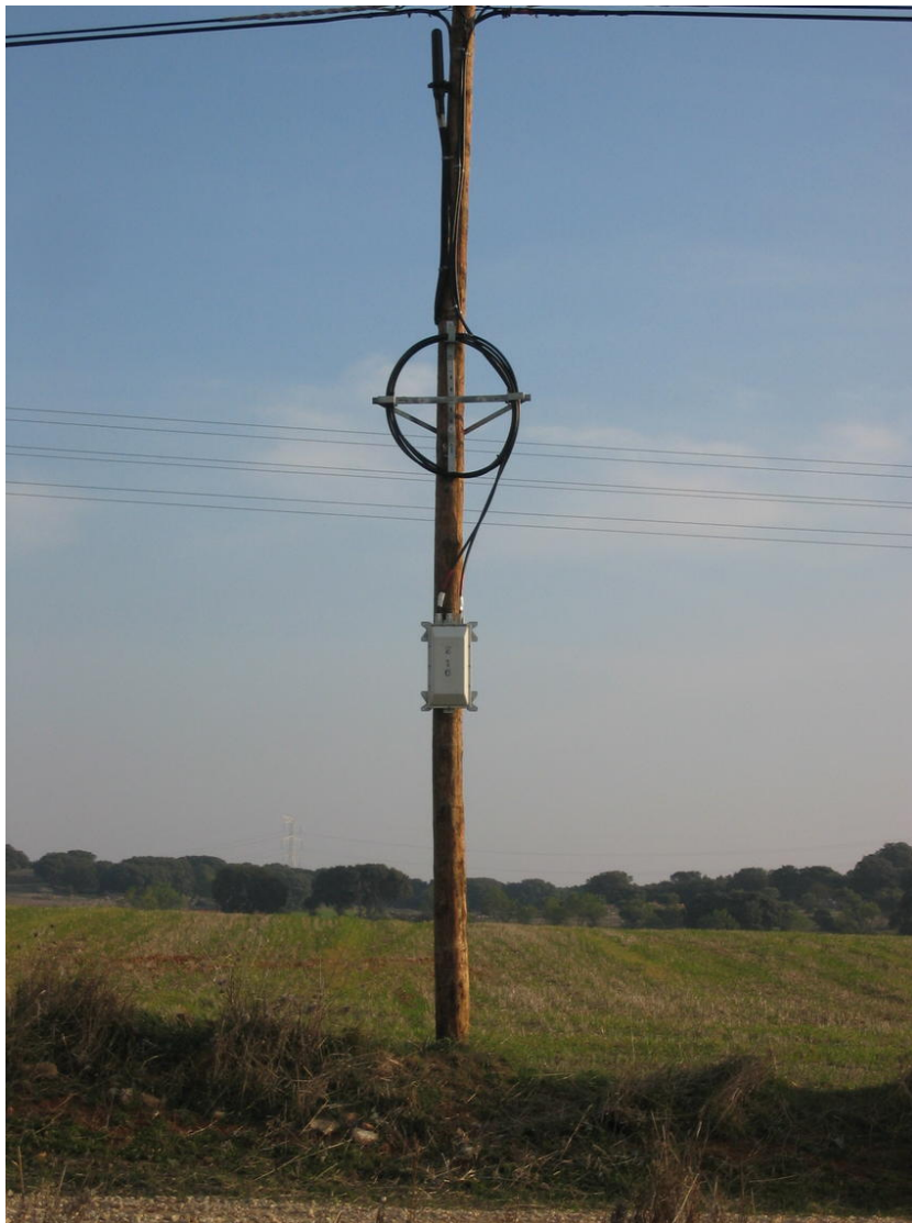
Figura 3: Wooden mast with a connection box that houses the soldering
